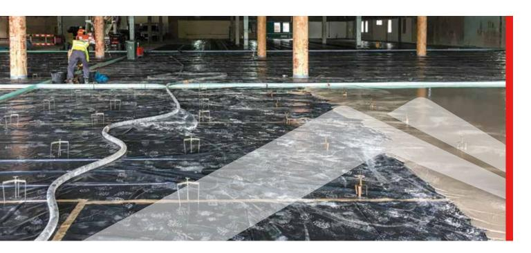
Gypsol TS-15 screed is a revolutionary new anhydrite screed material. It is specially formulated to offer a strong and durable ultra-thin topping to a solid interior substrate, for example, in situ concrete or beam and block or precast concrete plank. Tested to BS 8204:1:2003 it meets the requirements for class A for impact resistance. Due to its ultra-thin depth, just 15mm minimum, TS-15 can be dried quickly allowing rapid return to service and application of finished floor coverings.
