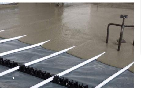
Due to self-compacting properties of Cemfloor Therm, it is specifically designed for use with underfloor heating systems.
